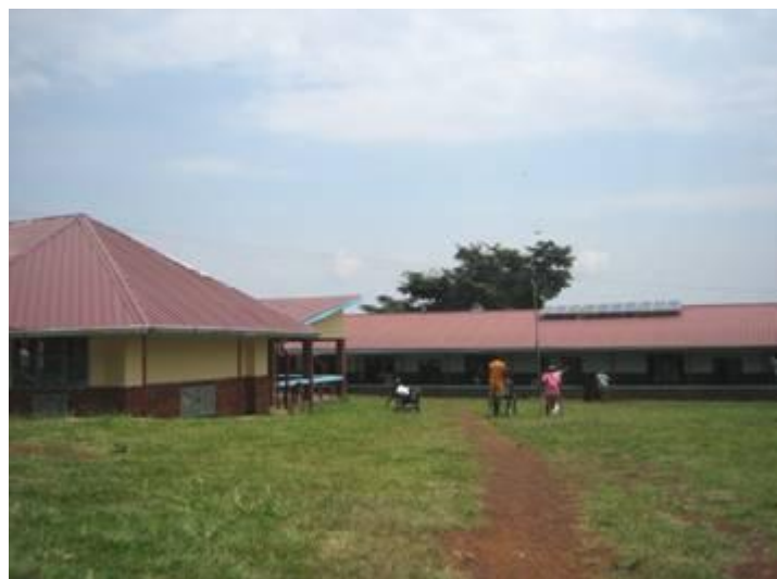
Rehabilitation center for children with disabilities, Masaka, Uganda.
